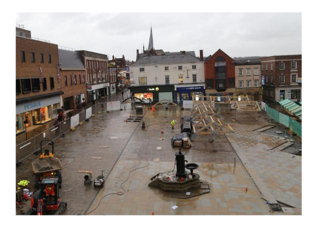
The first phase of town centre regeneration work in the upper section of Market Place is nearing completion – with the new yorkstone paving and restored and relaid cobbles now in place, helping to make the area more accessible.
